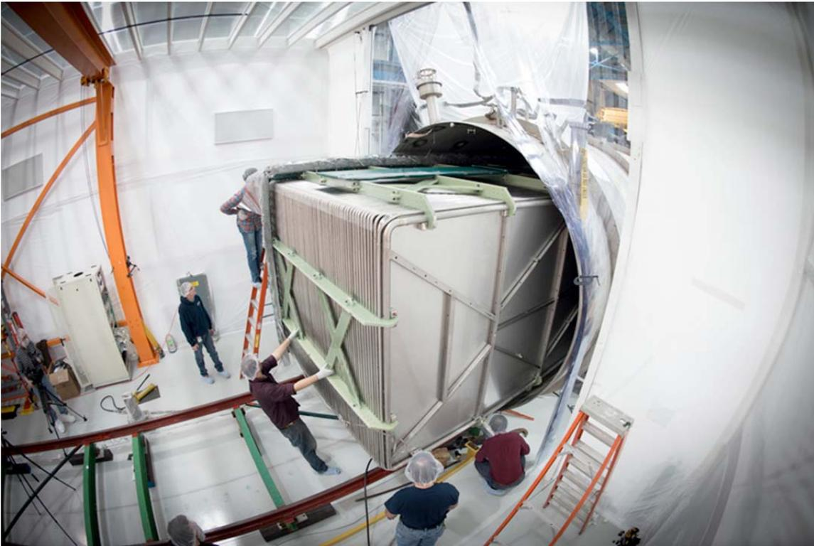
*Figure 4: Photograph of the TPC being installed into the cryostat.*
