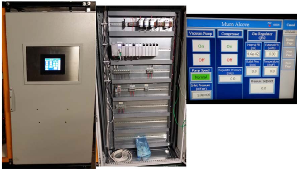
Figure 2: A photograph of the controls panel and touch pad.
