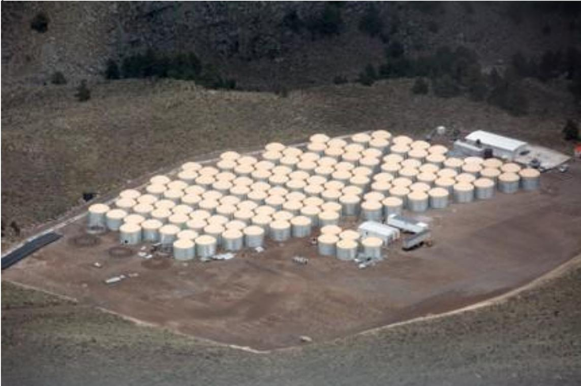
Figure 2 - Construction status of HAWC from early September 2013. In this image, there are 139 constructed tanks. The completed (as funded) HAWC detector will include 250 tanks. The platform was designed to accommodate 300 tanks.
