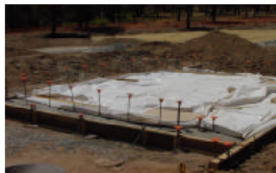
Dumpster Enclosure / Demo Wall May 24, 2002
