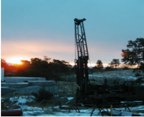
Geotechnical Drilling at Sunrise: TA-50-1, 12/15/01
