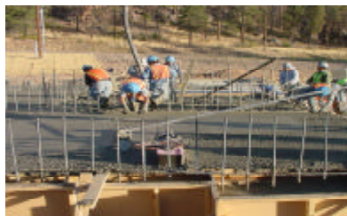
Final Top-Out - Placement #2 8:30 AM 5-23-02
