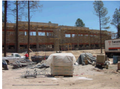
ESA-Division Office Building May 24, 2002
