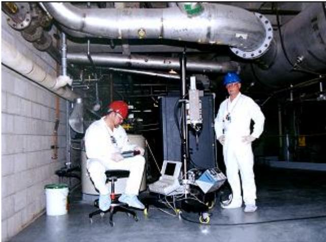
*Fig. 13. A large overhead duct is measured from below with a collimated Ge detector.*
