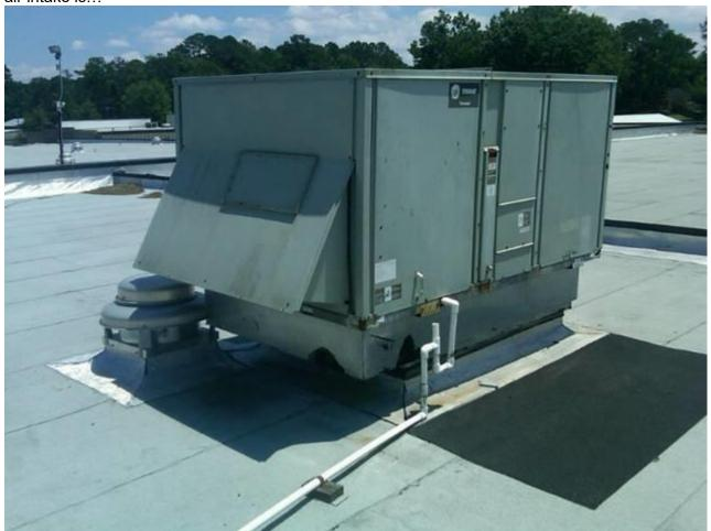
Nasty code violation unless exhaust fan is removed/sealed inside. Piping the condensate away instead of draining onto the roof is good but not offsetting.
