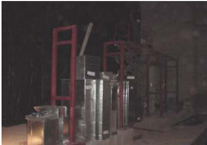
Installation of Christie Wall Frame in Primary EOC 1/23/03
