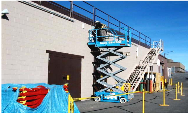
Installing Ethernet System at TA-50-01
