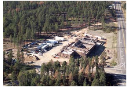
Aerial View of EOC Construction Taken At 2 nd Floor Concrete Completion
