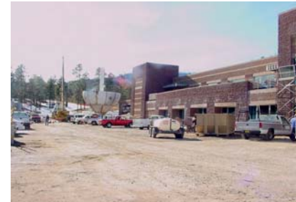
Installation Water Tower 1/23/03
